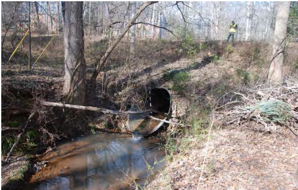
Photo 2: Downstream end of culvert looking northwest towards Merrydale Drive.
