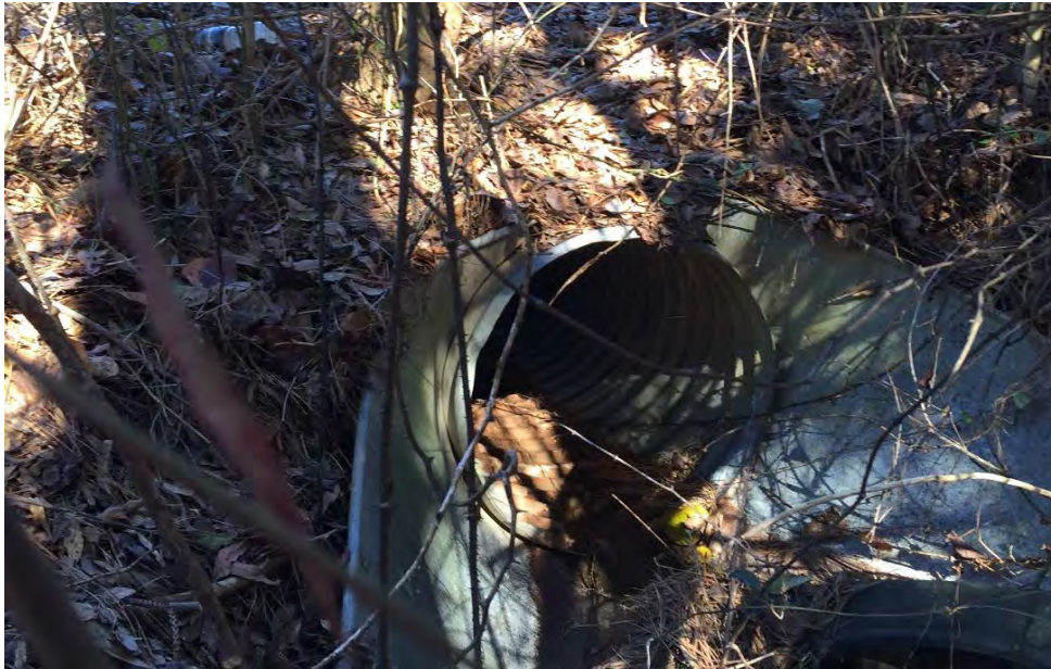
Photo 1: Upstream end of culvert looking North towards Millers Oak Way.
