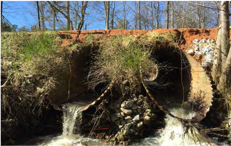
Photo 2: Downstream end looking South towards North Bend Court.
