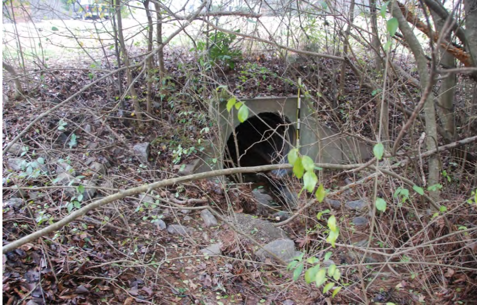
Photo 1: Upstream end of culvert.
