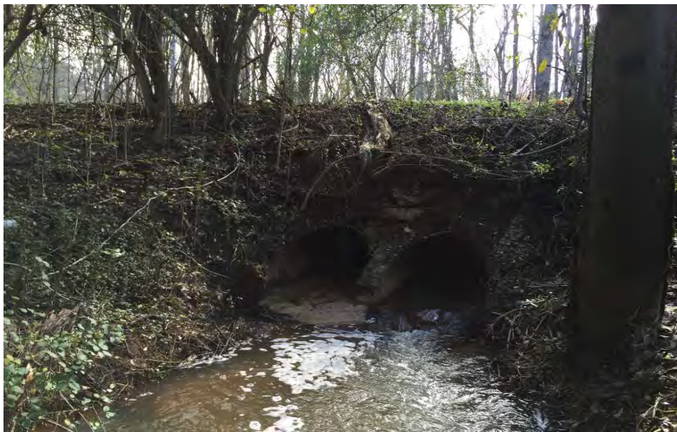
Photo 2: Downstream end looking East towards Greenfield Circle.
