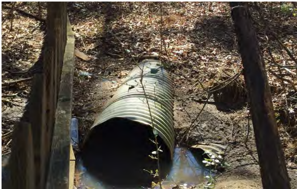
Photo 2: Downstream end looking North towards Millers Oak Way.
