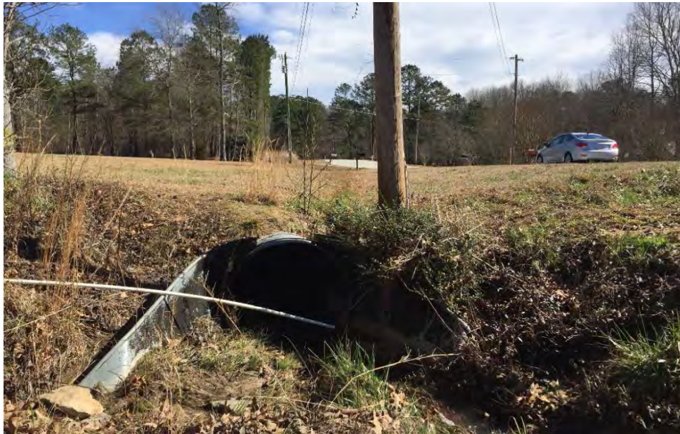
Photo 1: Upstream end of culvert looking East along County Line Court.
