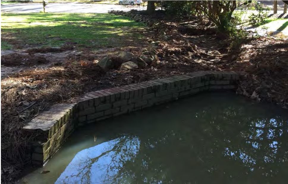
Photo 1: Upstream end of culvert looking South towards Deauville Way.
