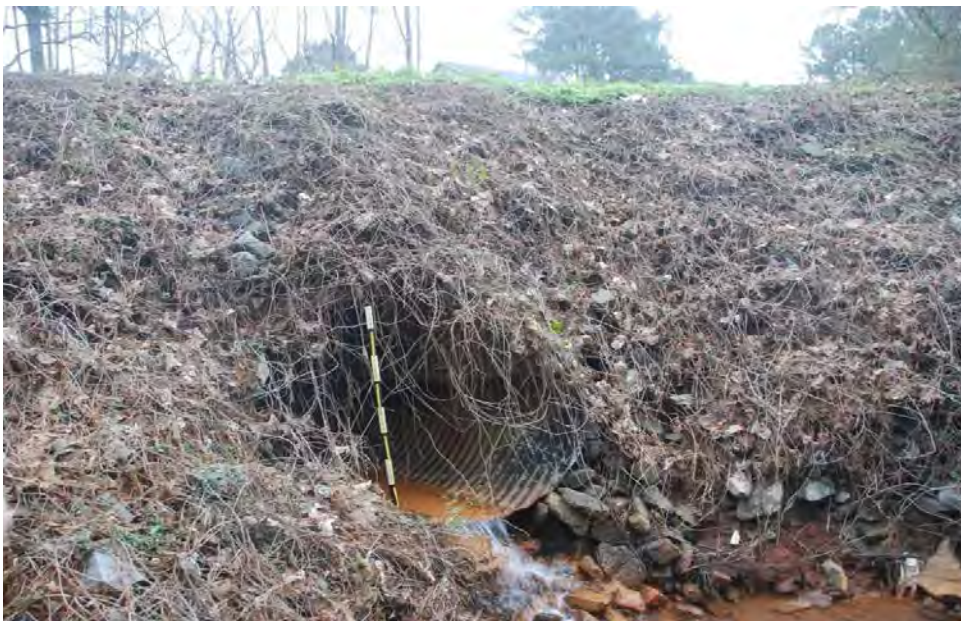
Photo 2: Downstream end of culvert.
