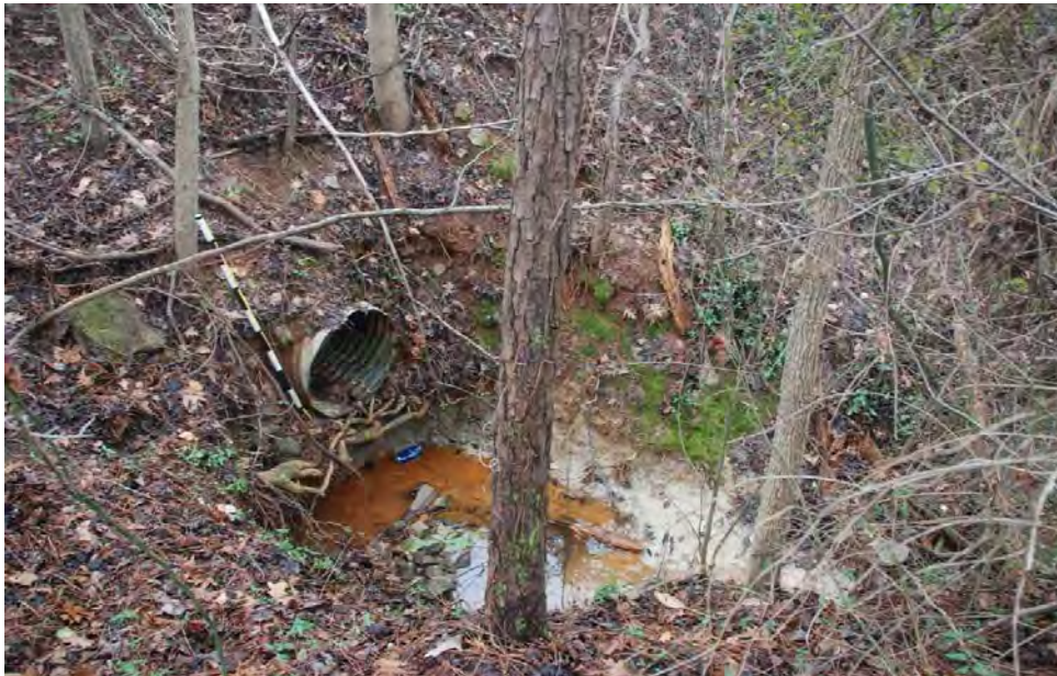
Photo 2: Downstream end of culvert.
