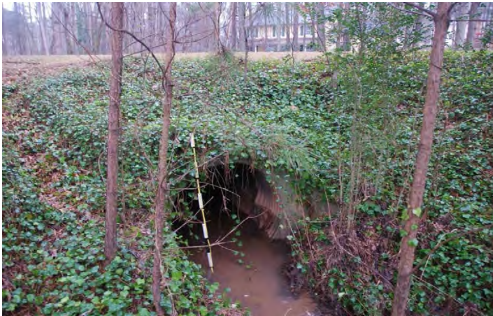
Photo 2: Downstream end of culvert looking North towards Kingswood Drive.
