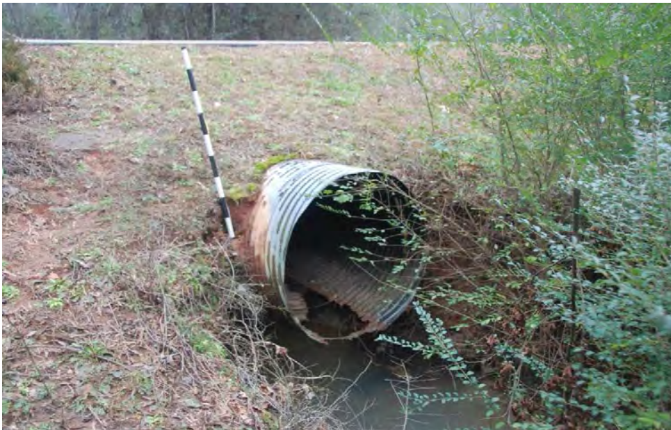
Photo 2: Downstream end of culvert looking North towards Cedar Trail.
