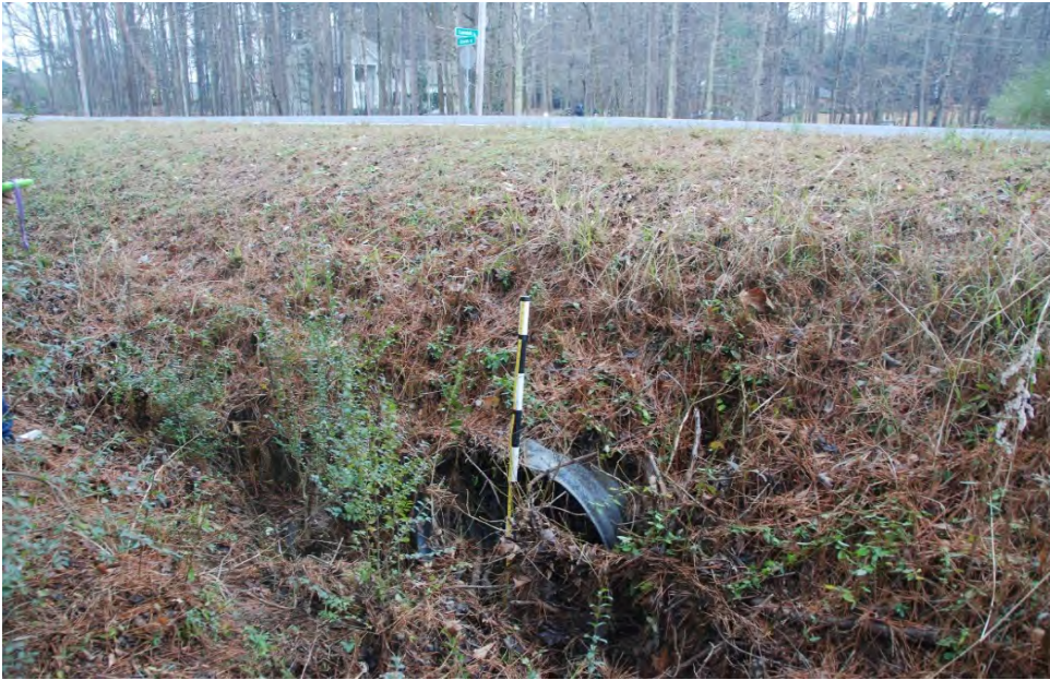
Photo 1: Upstream end of culvert looking South towards Graves Road.
