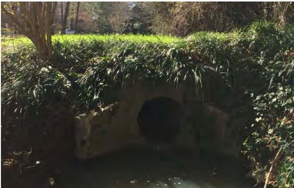
Photo 2: Downstream end looking West towards Deauville Way.
