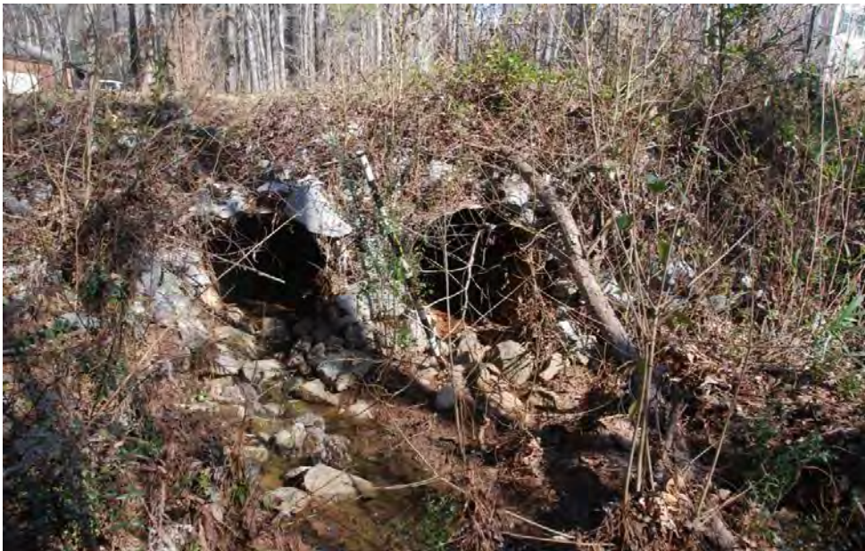
Photo 2: Downstream end of culverts
