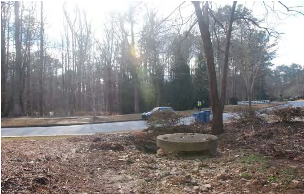
Photo 2: Upstream inlet looking West towards Old Ivy.
