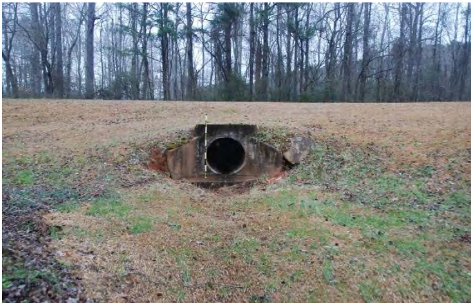
Photo 2: Downstream end of culvert.
