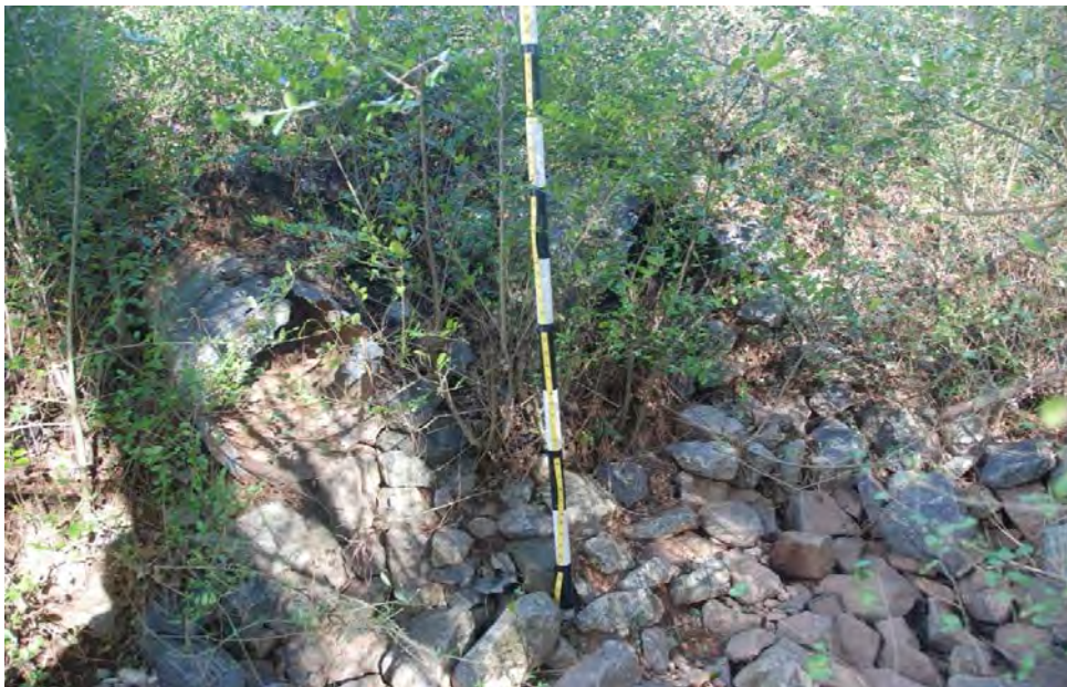
Photo 2: Downstream end of culverts.
