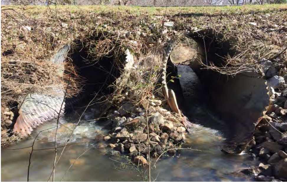
Photo 1: Upstream end of culvert looking East towards Inman Road.
