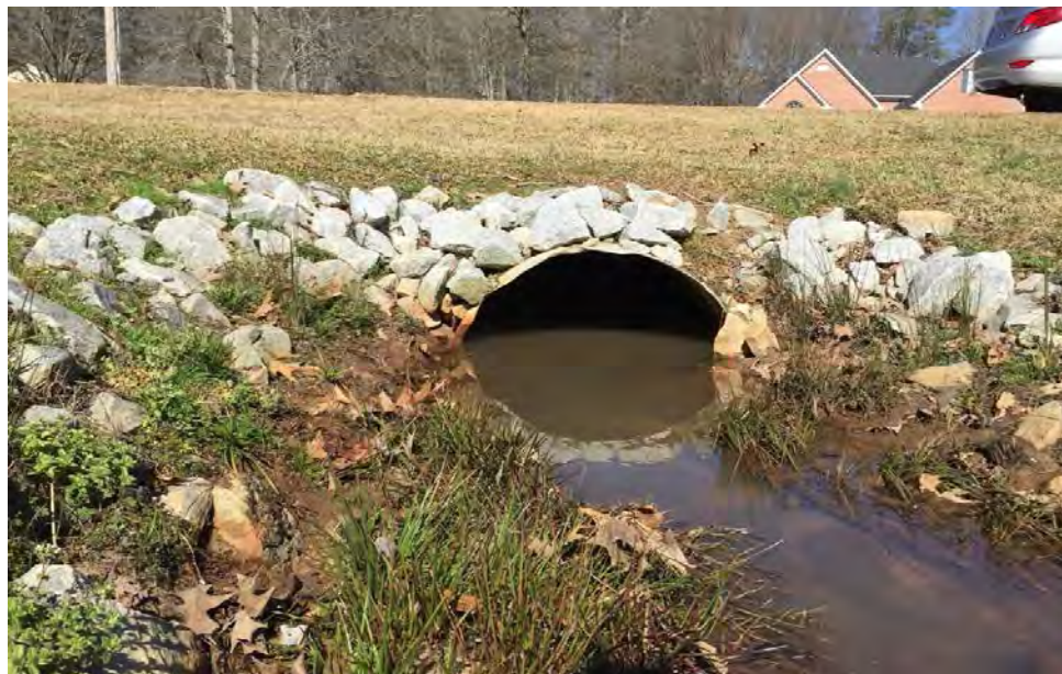
Photo 2: Downstream end looking North towards County Line Court.
