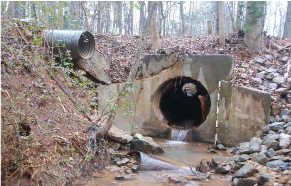
Photo 2: Downstream end of culvert looking West towards Derby Drive
