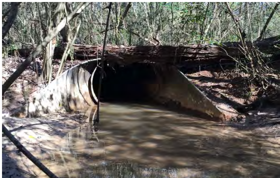
Photo 2: Downstream looking South towards North Bend Court.
