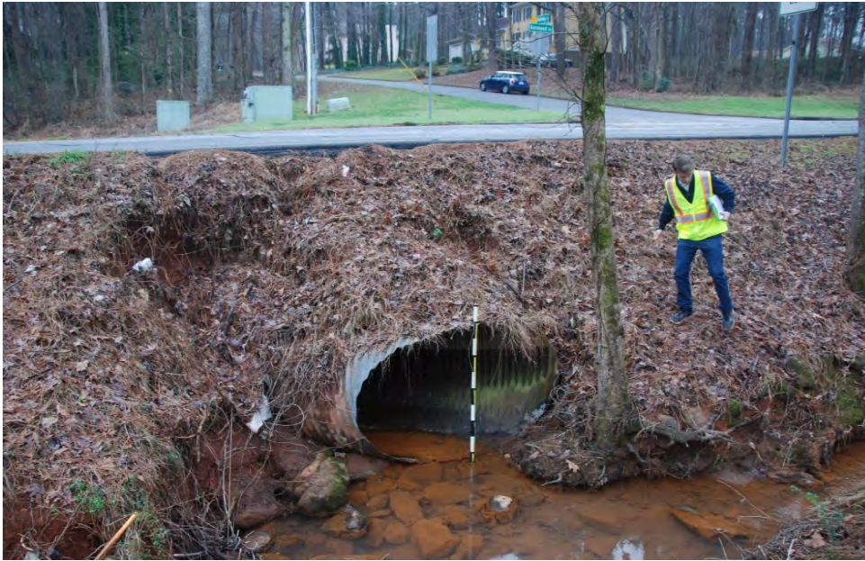
Photo 1: Upstream end of culvert looking South towards Kenwood Road.
