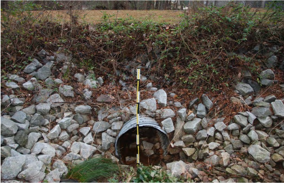
Photo 1: Upstream end of culvert looking North towards Oak Street.
