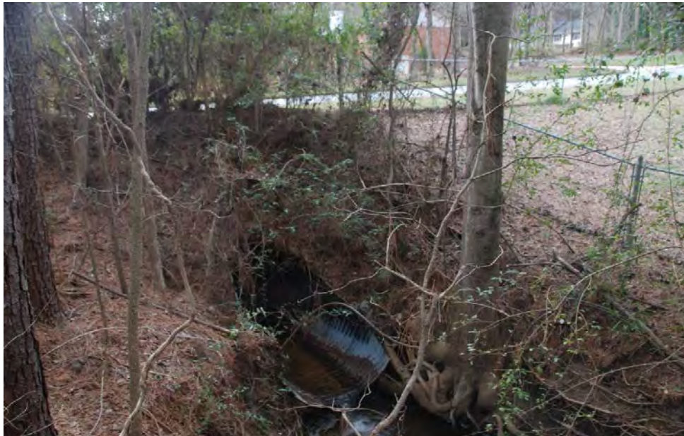
Photo 2: Downstream end of culvert looking northeast towards Brockton Court.
