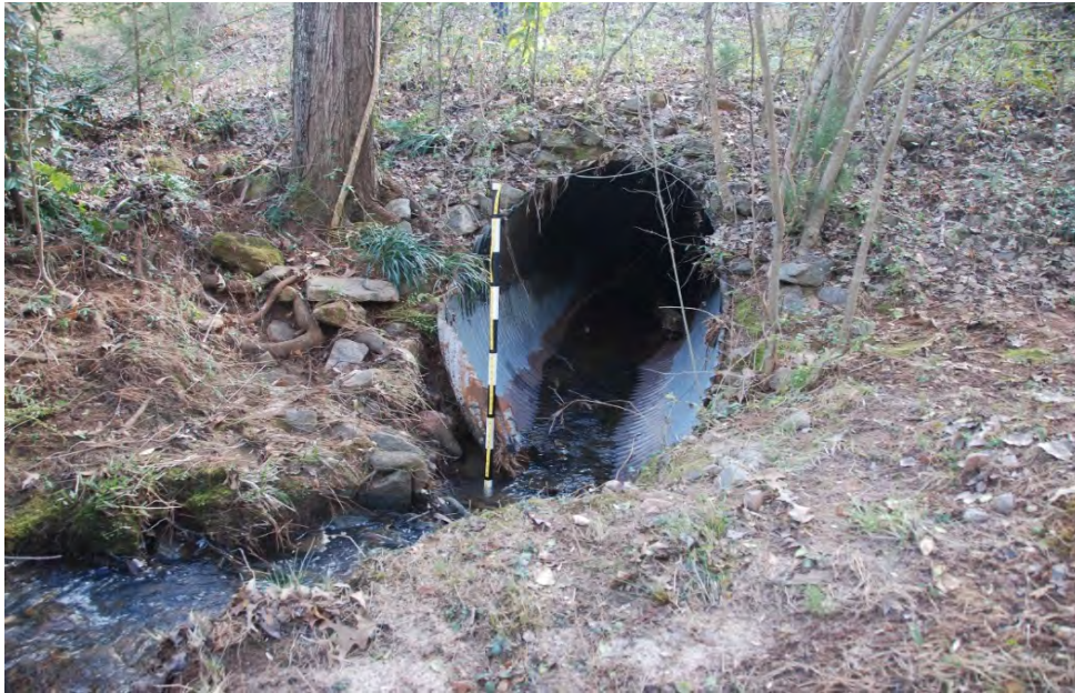
Photo 1: Upstream end of culvert.
