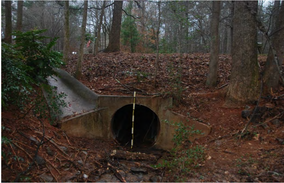
Photo 1: Upstream end of culvert.
