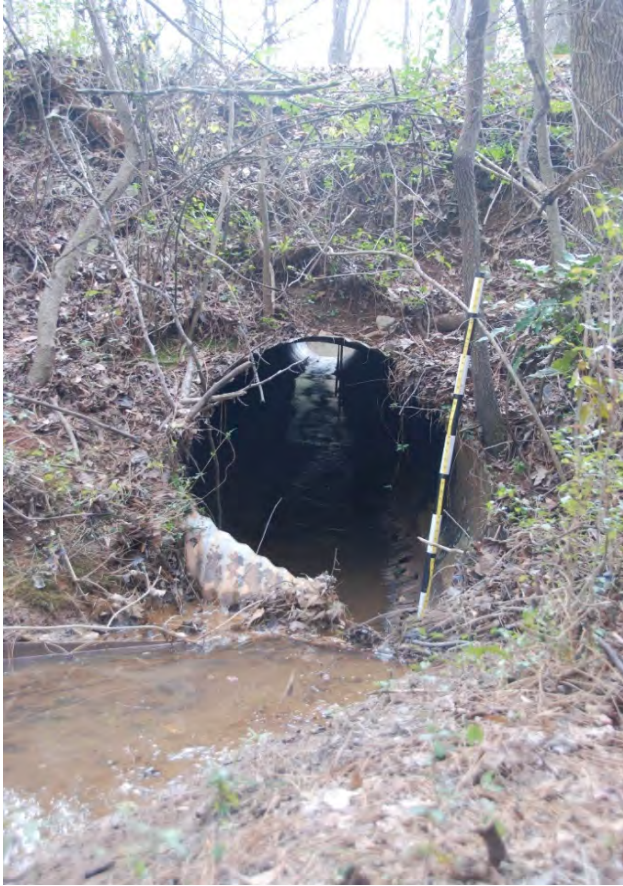
Photo 1: Upstream end of culvert.
