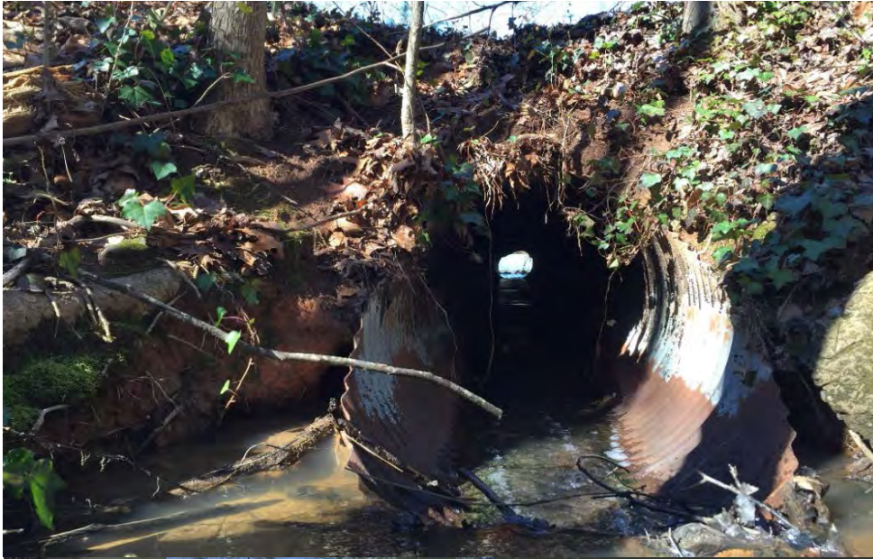
Photo 1: Upstream end of culvert looking West towards Greenfield Circle.
