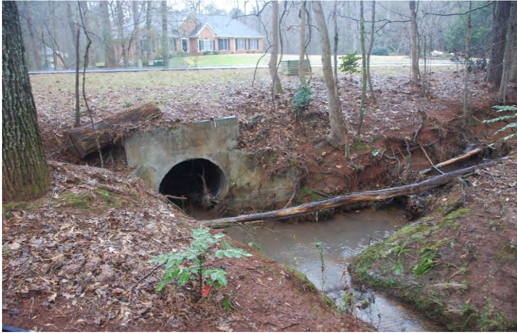
Photo 1: Upstream end of culvert looking East towards Derby Drive
