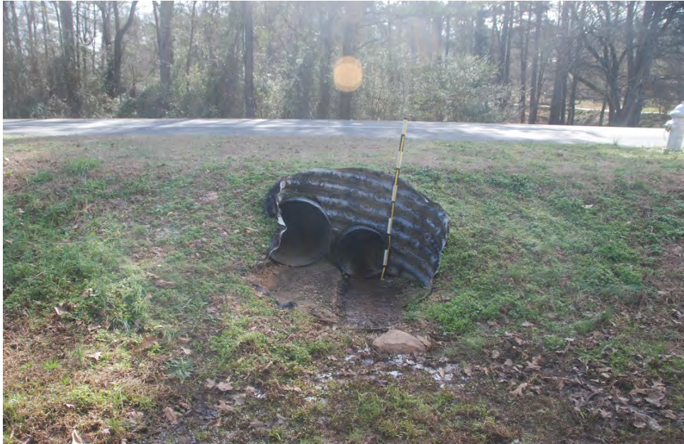
Photo 1: Upstream end of culverts looking South towards Hilo Road.
